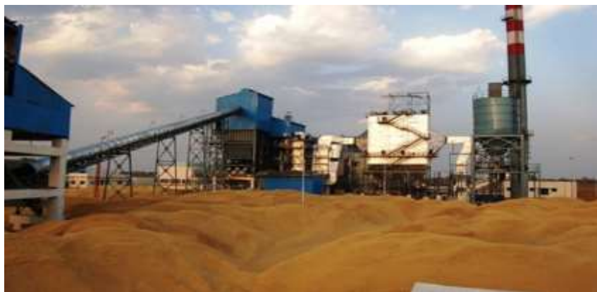
10 MW Biomass Power Project, Gadchiroli Distt. (Maharashtra State)
