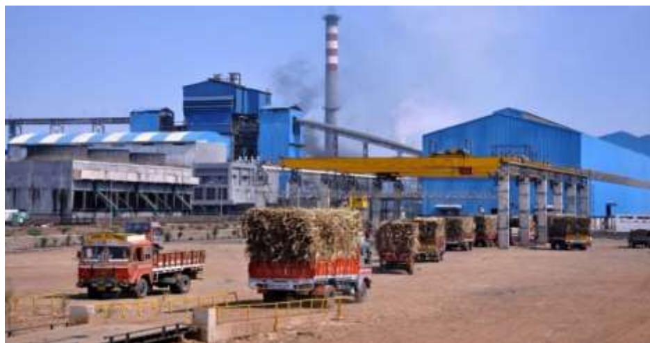
30 MW Bagasse Cogen project at a Sugar Mill in Maharashtra
